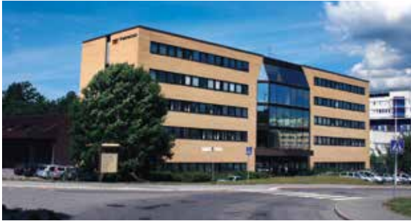
TERCO headoffice and factory outside Stockholm, Sweden
