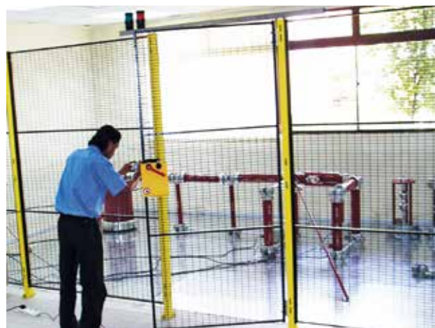
Installation of Safety Fence
